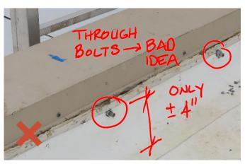
It is recommended to connect to the substrate above the roofing or as high as possible to avoid water, snow, and ice build-up near the attachment location.
